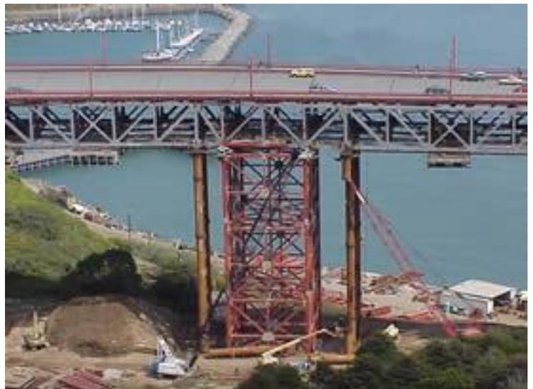
Fig. 10, *New support tower under construction*
