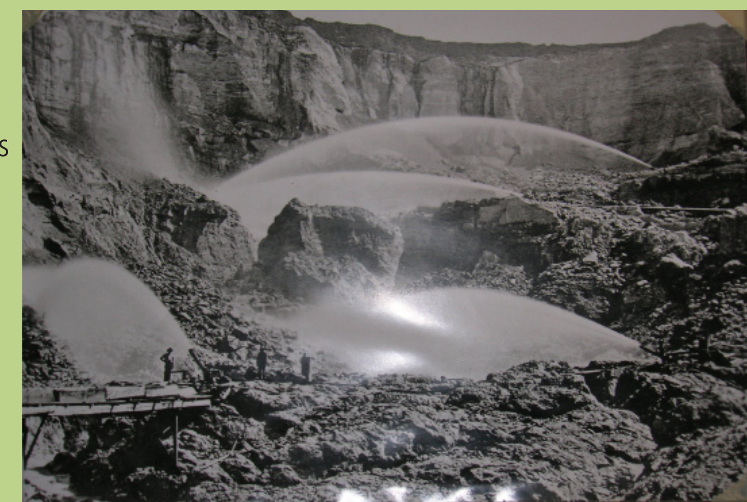
Hydraulic mining in the foothills of the Sierra Nevada. Photo from Sutter's Mill Museum.
