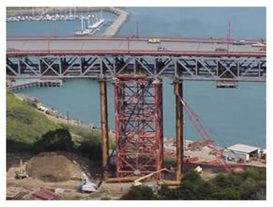
Fig. 10, New support tower under construction
